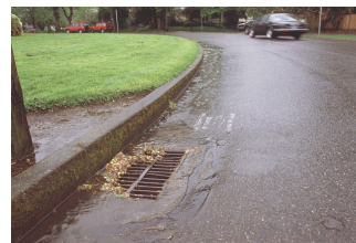
Yard waste flowing into a storm drain
