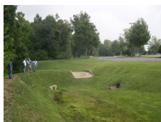
Dry Detention Basin
